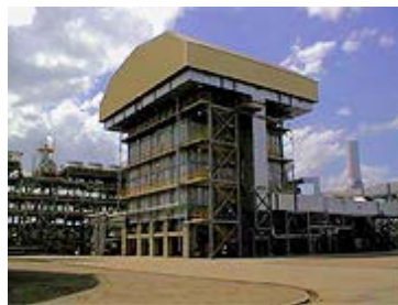
Trinidad steam reformer.
