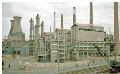
The Methanol plant at ICI in Billingham, September 1970.
